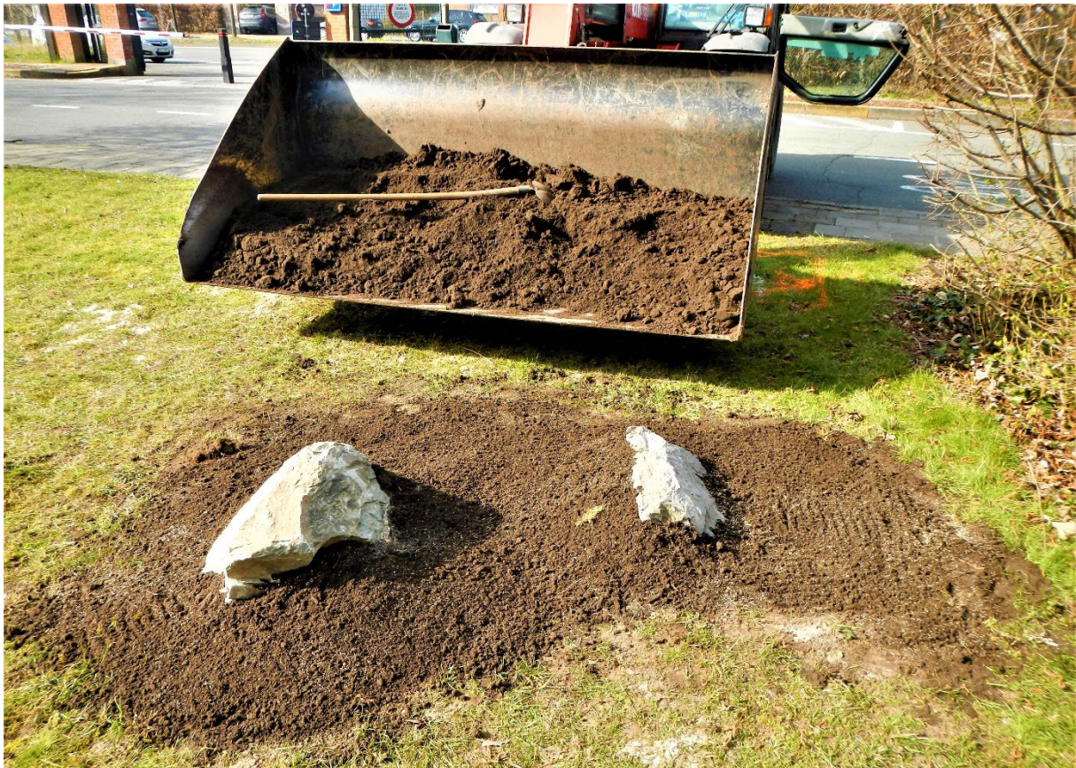
Figure. Installation of Rock Garden blocks on Campus De Sterre.
